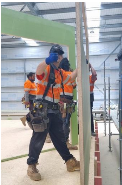
Once all Panels have been squared off, and the dimensions are all correct, then the panels are tightly secured to the floor using bracing brackets. These ensure the Panels are securely attached to the floor, providing maximum rigidity.
