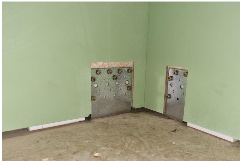
Once all Panels have been squared off, and the dimensions are all correct, then the panels are tightly secured to the floor using bracing brackets. These ensure the Panels are securely attached to the floor, providing maximum rigidity.
