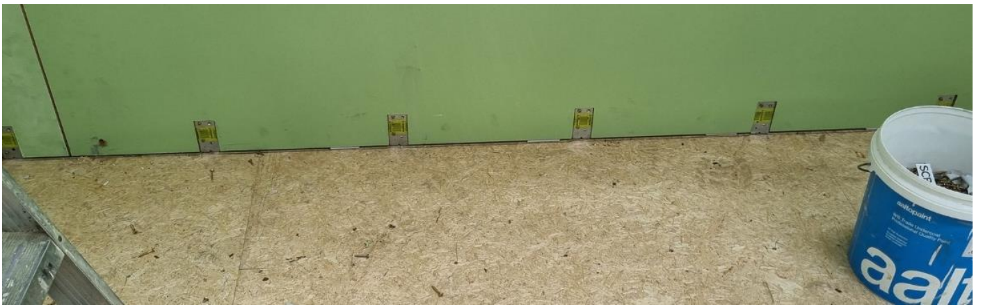
Once all Panels have been squared off, and the dimensions are all correct, then the panels are tightly secured to the floor using bracing brackets. These ensure the Panels are securely attached to the floor, providing maximum rigidity.
